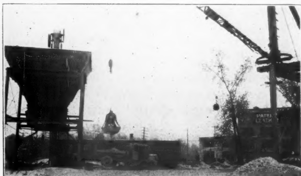
Loading Trucks with Derrick
